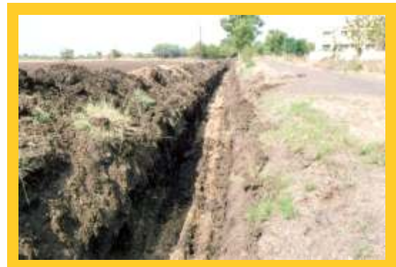
Field Channel for Safe disposal of excess runoff
